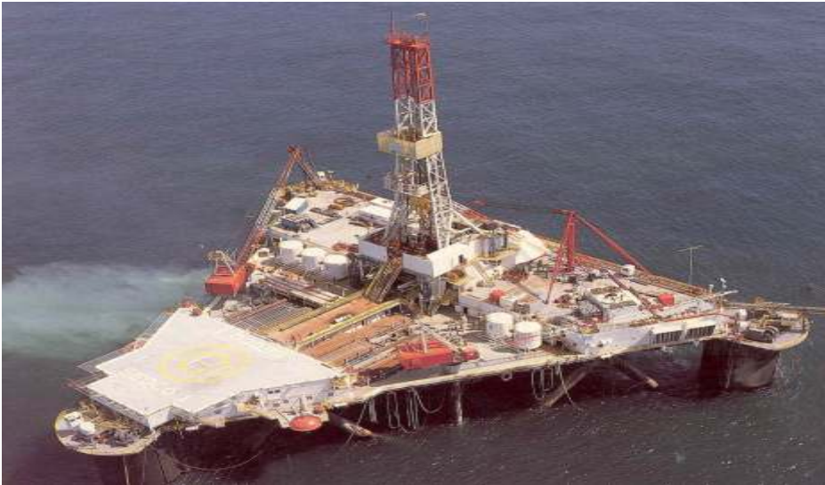
An offshore Oil Drilling Ring in the NDR
